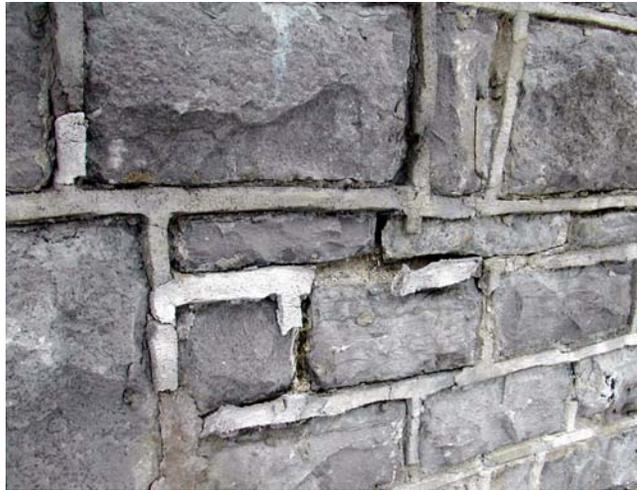
Figure 1 Frost damage in a wall with a dense repointing mortar
